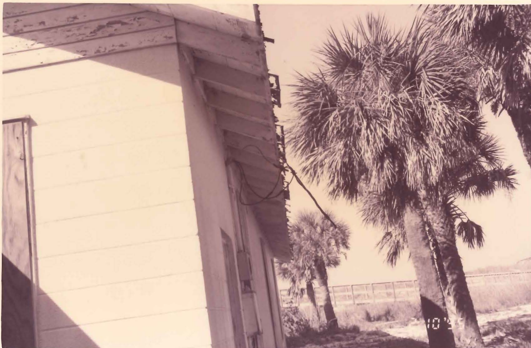
Close-up of open wood rafters on northern elevation
