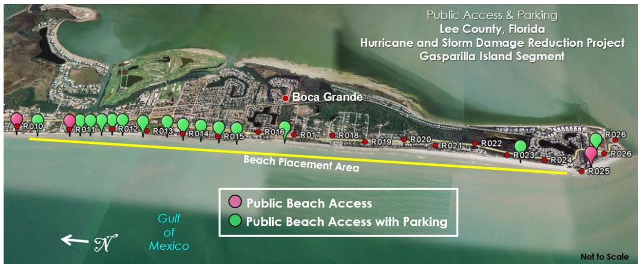
Figure 1: Shoreline image for subject area depicting FDEP R-monuments and public access points
