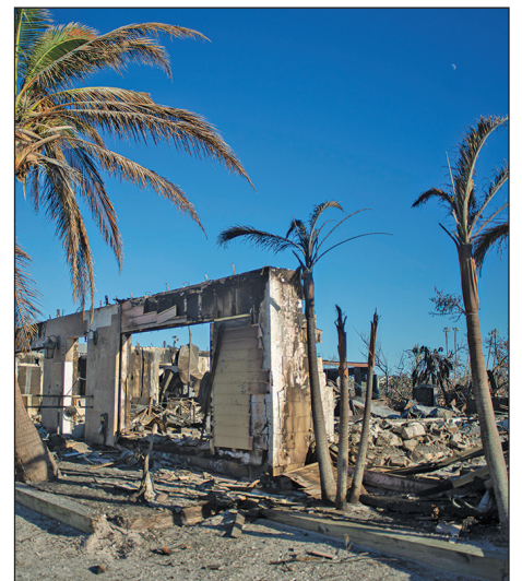
At right, the restaurant in ruins after the natural gas explosion at South Beach Bar & Grille during Hurricane Ian. Photo by Dusty Hopkins
